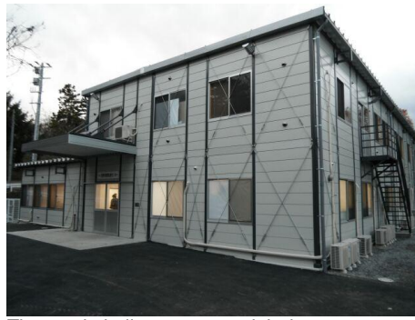
The newly built temporary night-time emergency medical centre in Ishinomaki; a steel-framed two story temporary building. ©JRCS
