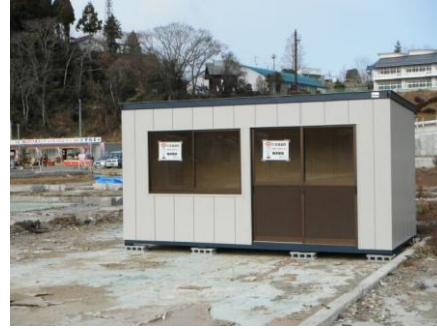
A temporary bus stop in Minamisanriku, protecting the users from strong coastal winds and snow as the temperature stays below zero Celsius in this region. ©JRCS
