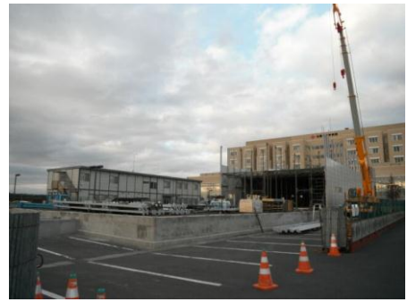
Construction under way in the former parking lot of Ishinomaki Red Cross Hospital. ©JRCS
