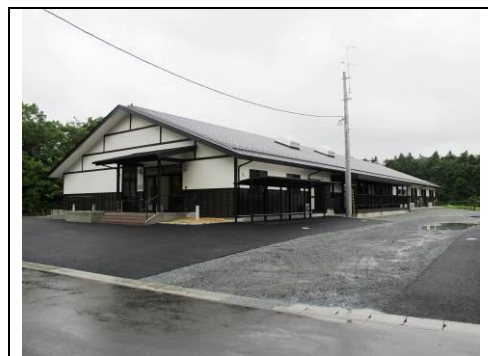
The first public housing built under recovery support project in Soma, Fukushima ©JRCS,.
