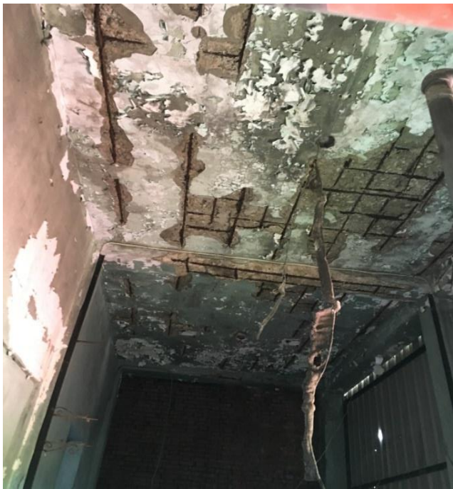
The ceilings, columns, and beams in the attached buildings of the tennis court were severely damaged and were reconstructed with reinforced concrete after demolition
