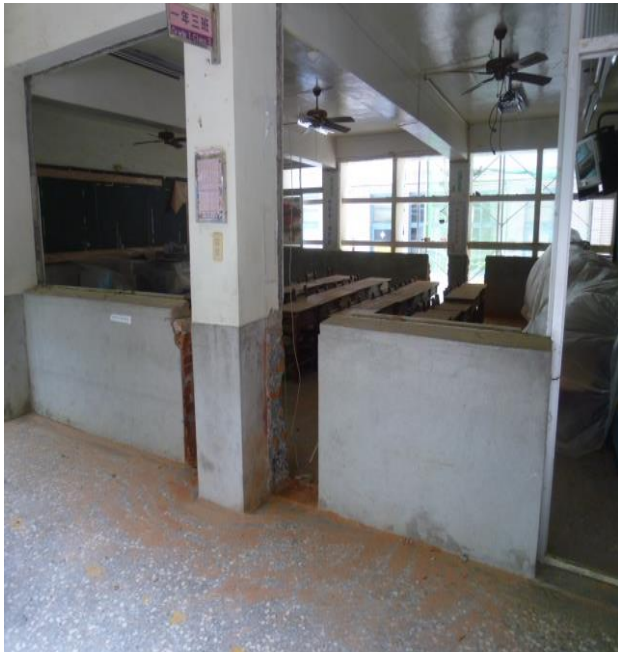
Classroom building suffered structural damage due to the short column effect
