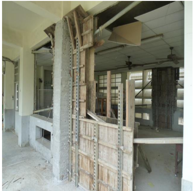
Reinforced through the wing wall method
