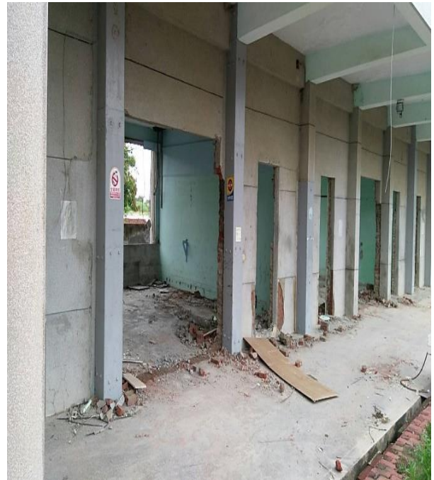
North wing classroom pillars awaiting demolition, as the original steel reinforcements have cracked
