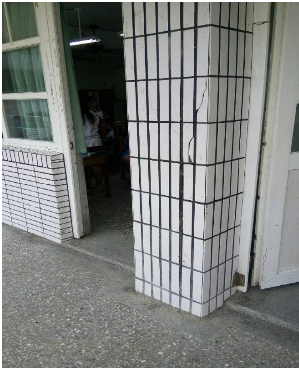
Pillars in the front of the classrooms had cracked and were reinforced by column jacking. Accountability plaque recognizing your society's contribution
