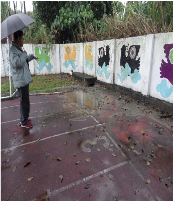
The PU runway had collapsed after the quake, collecting water
