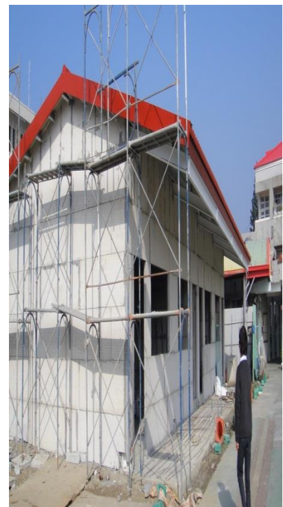
West wing classrooms severely damaged. After demolition, the structure was reconstructed using steel structures and light partition walls to be safe and shock-resistant
