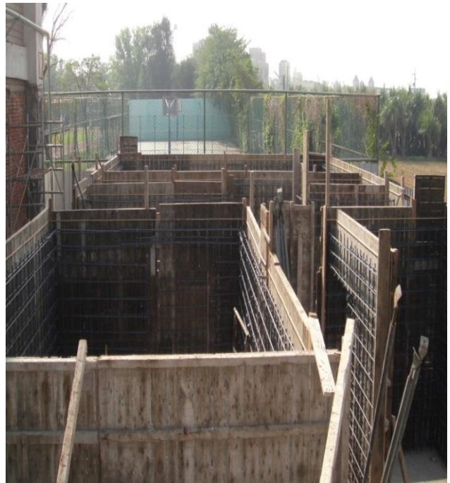
The ceilings, columns, and beams in the attached buildings of the tennis court were severely damaged and were reconstructed with reinforced concrete after demolition
