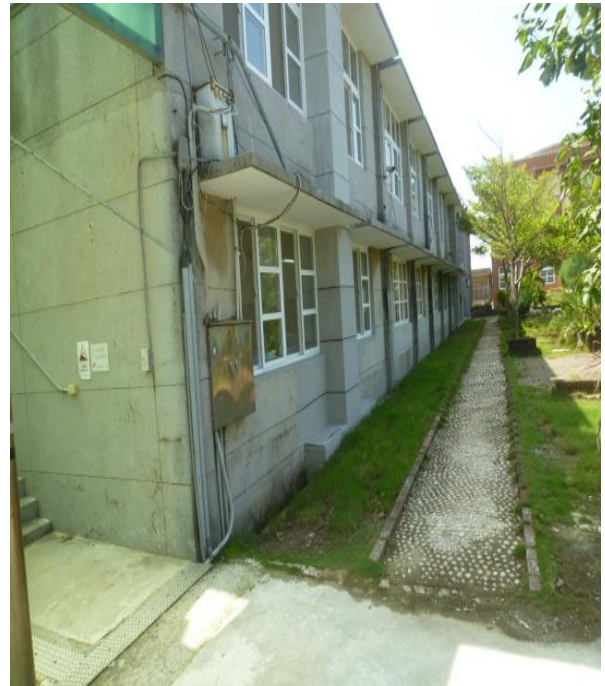
Pillars in the back of the classrooms were reinforced by column jacking. The original wooden window frames were replaced with PVC frames
