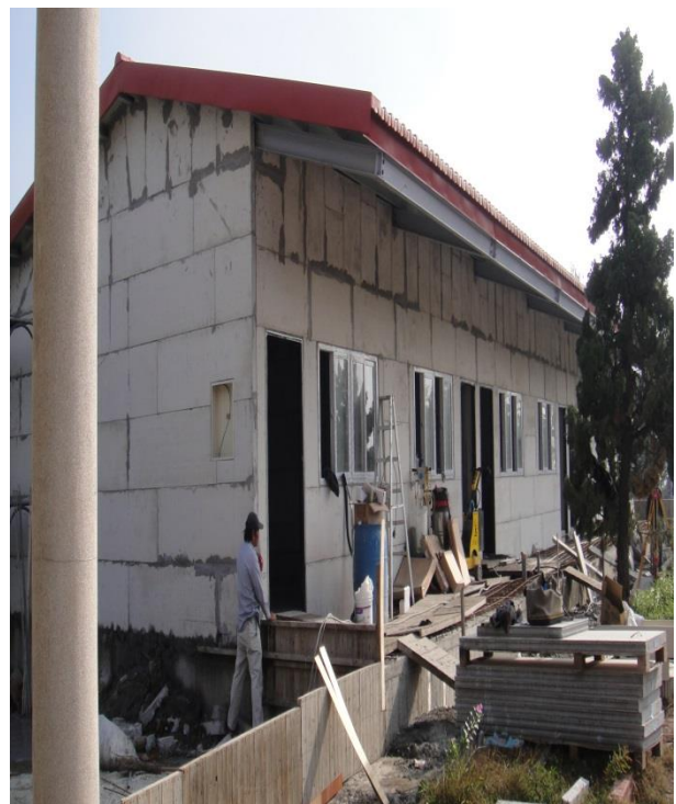
After demolition and importing German light partitions, this building is now shock and fire-resistant
