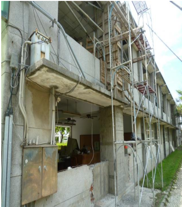
Pillars in the back of the classrooms were reinforced by column jacking. The original wooden window frames were replaced with PVC frames
