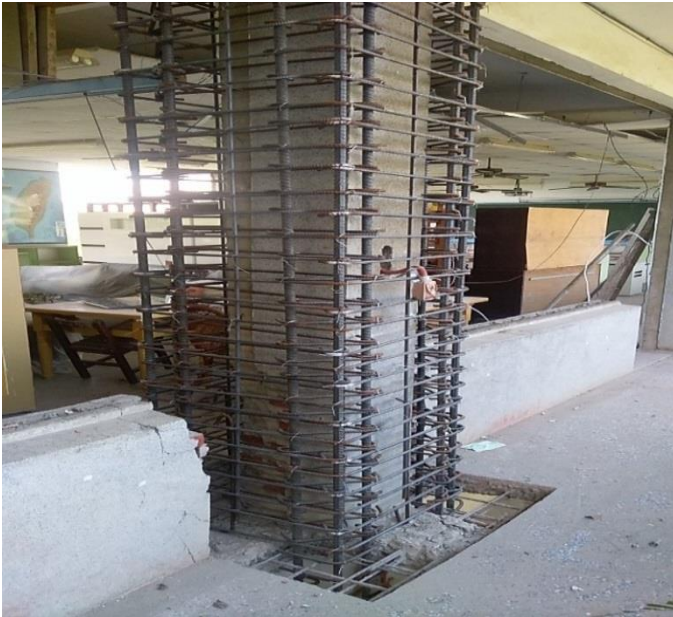
Shorter walls and windows within classrooms are the most prone to damage from the short column effect. Pictured on the left are wing walls, on the right is column jacketing, which are two methods of making classroom structures more earthquake-resistant and safe.
