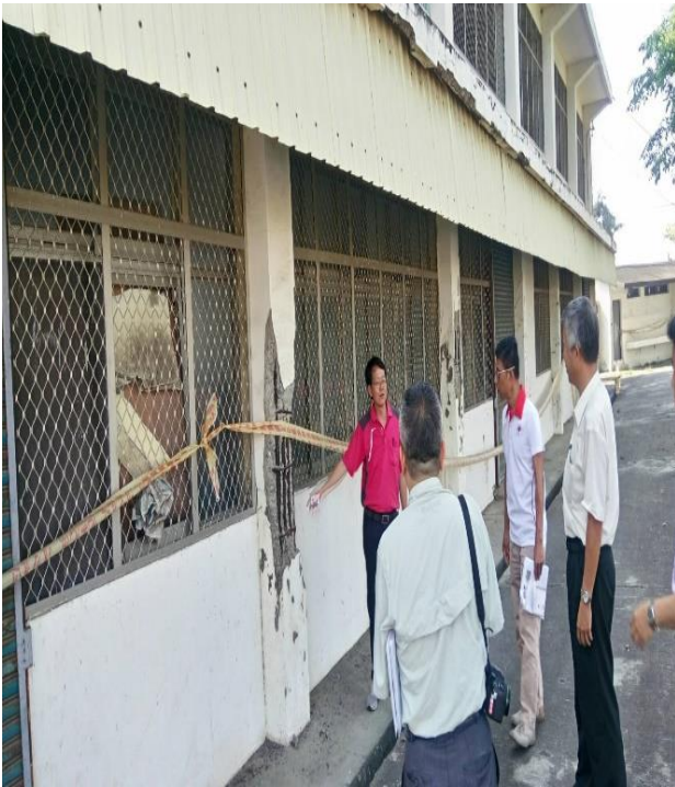
The beams and columns in the industrial arts classroom were severely damaged. Demolition and reconstruction were deemed necessary after structural safety assessment
