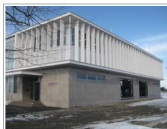
building with the storehouse in the first floor of the building. © JRCS
