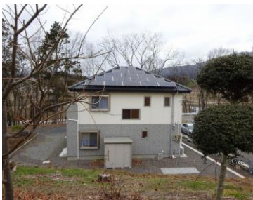
Installation of the solar power systems in Iwate. ©JRCS.
