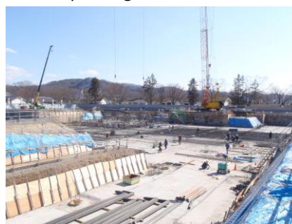
Fukushima Red Cross Hospital is under construction in February 2017. © JRCS
