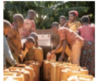
Residents waiting in line at the newly installed village water supply point
